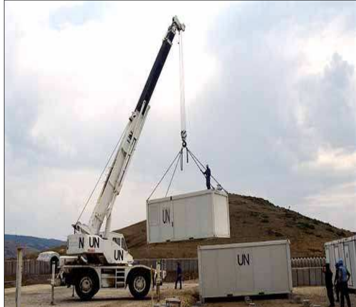
UNPREDEP Peacekeepers, part of the Indonesian Engineering platoon, use containers to construct a new observation post along the Yugoslav Border (1996). (UN Photo #187928)
