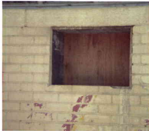
Figure 2: Outside wall of MovCon warehouse
