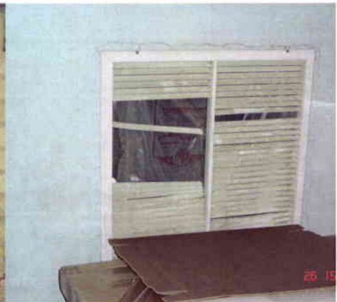
Figure 3: Inside wall separating Supply and MovCon warehouses
