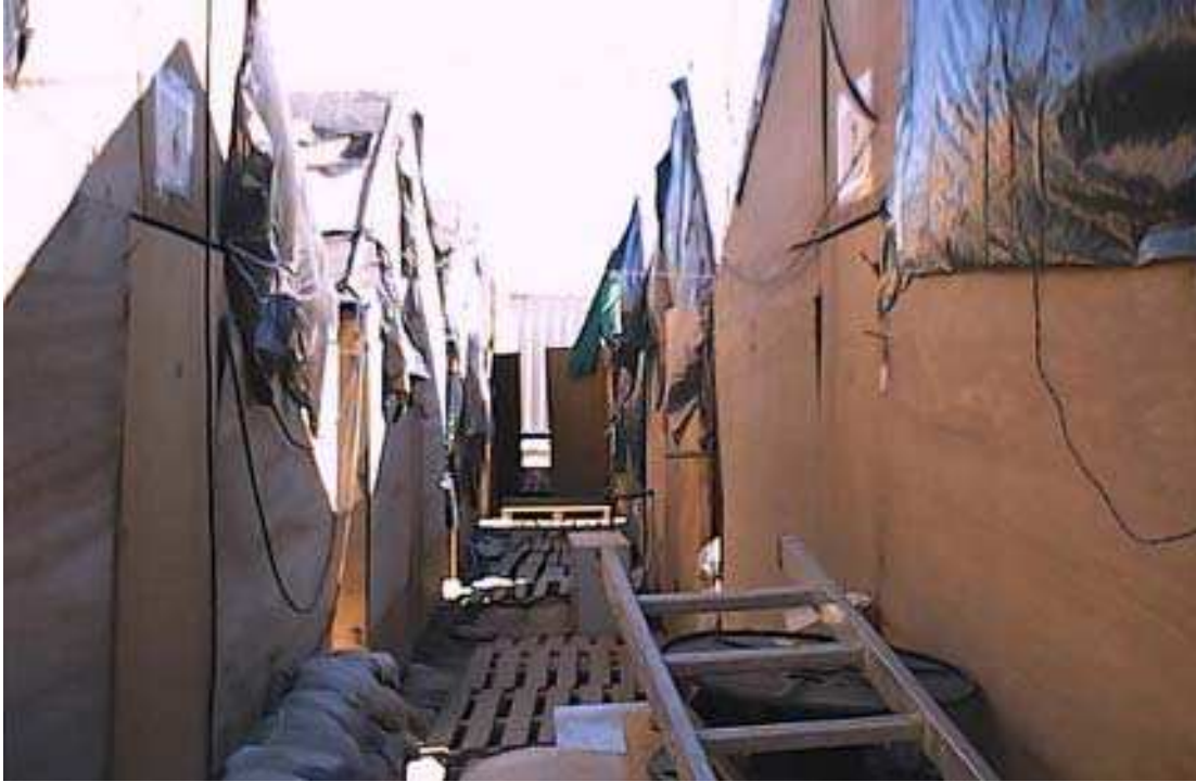
Proper planning includes common safety and mitigation considerations, such as adding fire breaks and protective measures between expeditionary shelters. Here SEAHUTs provide little protection or access during emergencies.
